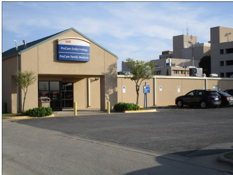
Parcel Two 315 North Golder Avenue
