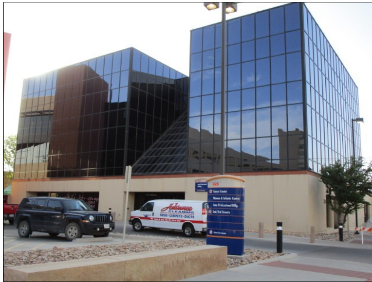
MCH Professional Building 318 North Alleghaney, Suite 201 Odessa, Texas
